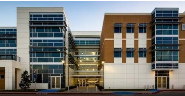
North Allied Health & Natural Science Building
